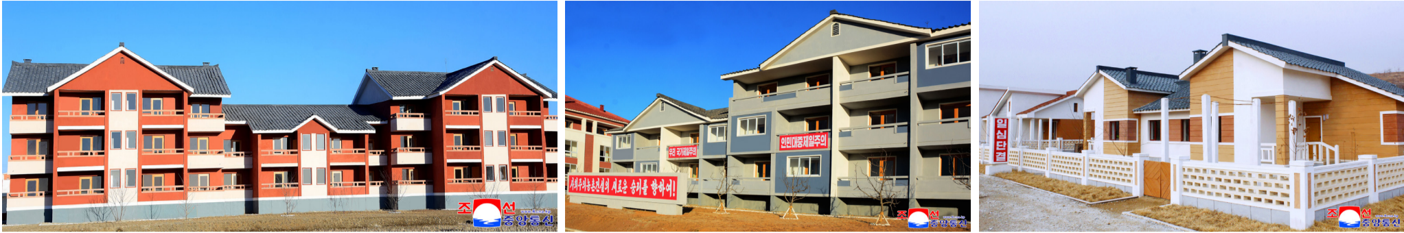
New houses built in Songhan-dong and Sonsang-dong of Sinuiju City, North Phyongan Province, and in Sanbuk-ri of Suan County, North Hwanghae Province.
