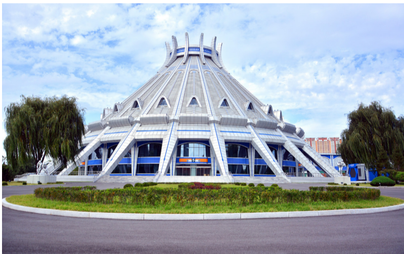
A view of the renovated Ice Rink.
