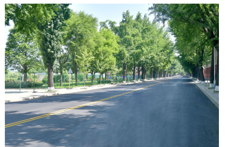
The renovated riverside road in Songyo District.
