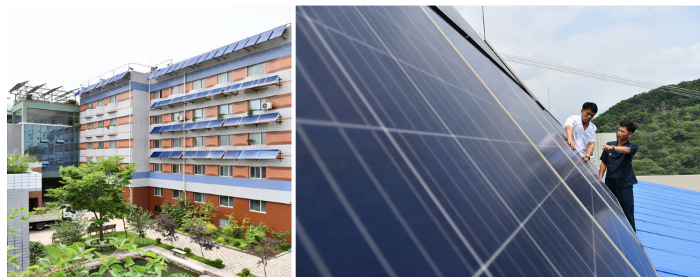
The management bureau derives considerable benefits from its solar energy generation system and air-conditioning system based on geothermal energy.
